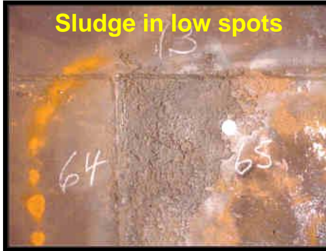
Sludge in tanks
