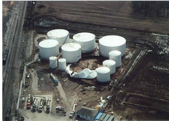
Quickly resulted in complete tank collapse... ..
